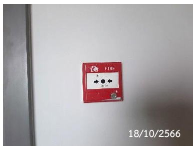
Fire Alarm Manual Station
