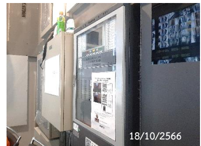
Fire Alarm Control Panel
